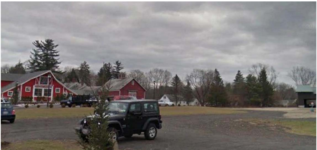
Bottom: View of the site facing east, including the recently rehabilitated barn that is now Atkins Market.
