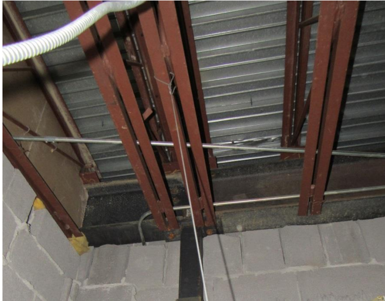
Figure 4 – Steel framing appears to be in excellent condition
